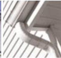
Soffit, Fascia and Rainware
